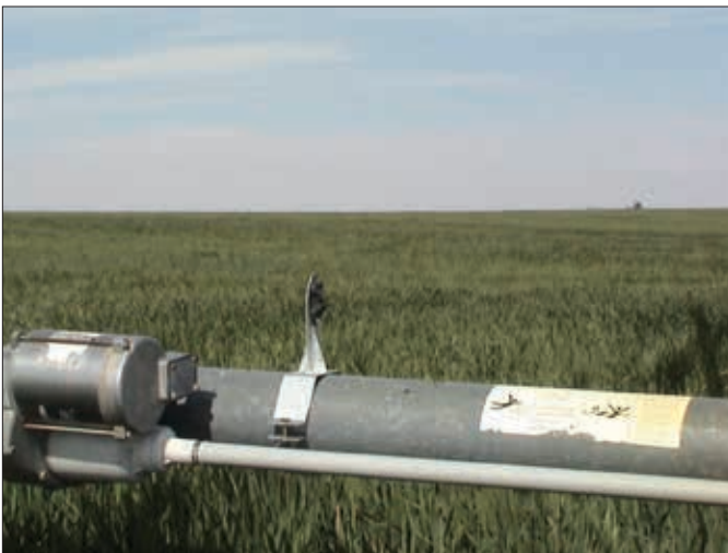
►A wire clamp with an insulator is fixed to the tower brace pipe and works to stabilize the wire by keeping the wire from grounding on the pipe or on the drive motor.
